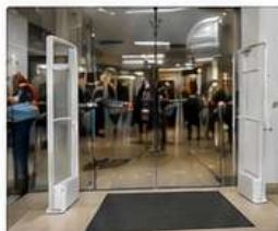
AM Antenna (Gate) Installation
