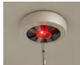
Alarm / Siren Installation
